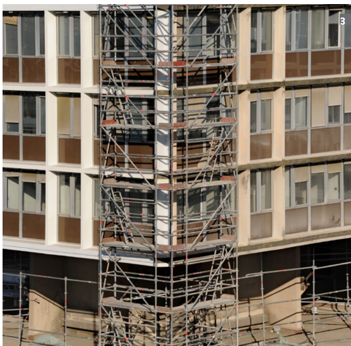
1 - Local confinement of columns using Foreva® TFC composite reinforcements
